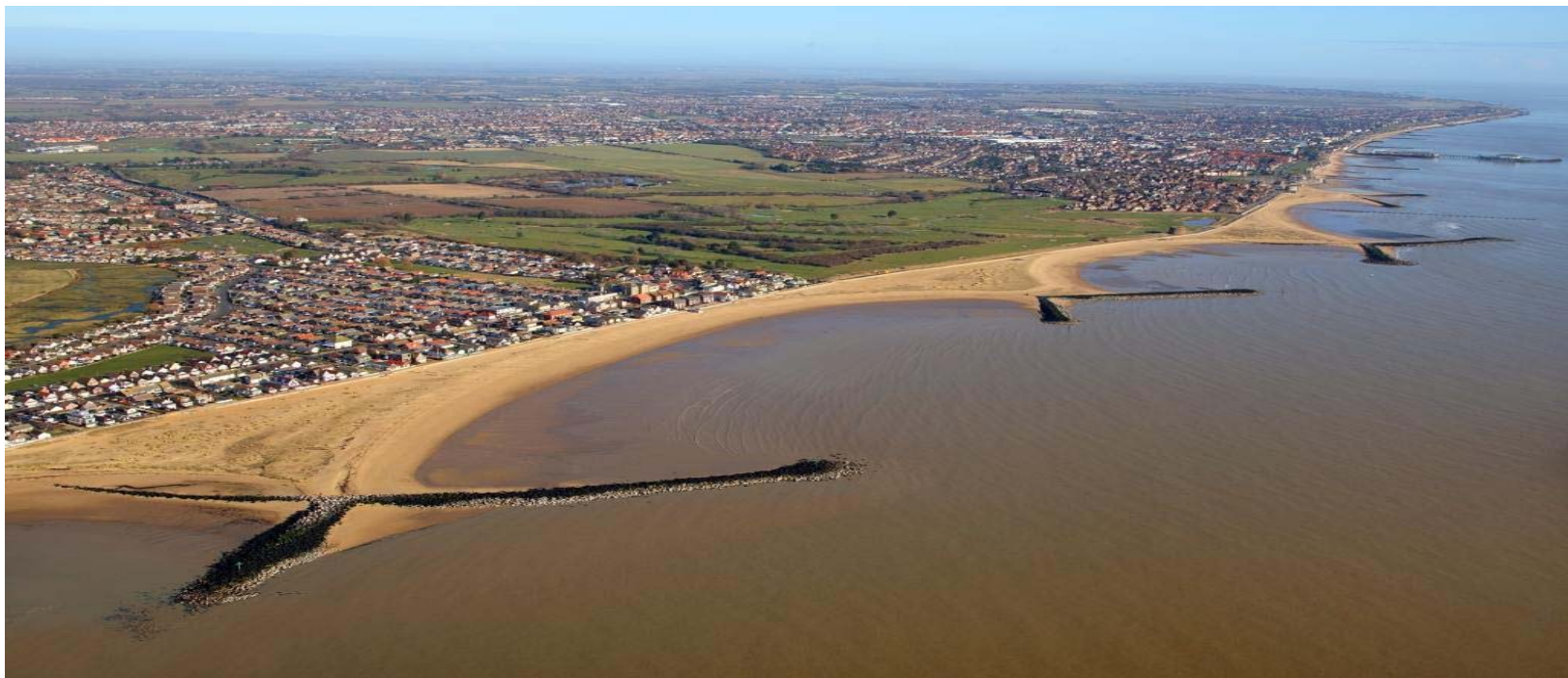
Fishtail rock groynes at Jaywick
